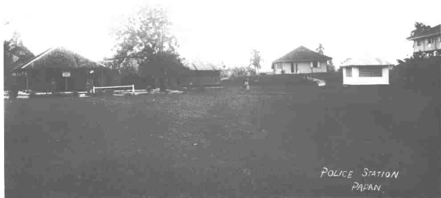
The Papan Police Station was built in 1886, and the married Police Quarters in 1888. The Police Station was demolished in early 2002.
